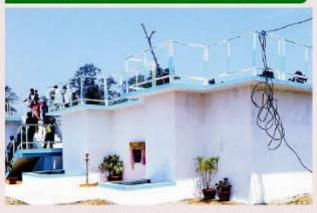
A Slow Sand Filter bed of capacity 2,70,000 ltr. per day with one Clear Water Reservoir (CWR) of 50,000 ltr. has been completed and commissioned by public of the area. INo. RCC Ring Well of 10 meter dia and dyke, as intake structure was also constructed .2 Nos. RCC surface tank of 1,36,000 ltr., and a sedimentation tank is also part of treatment unit.
