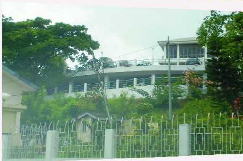
POLICE OUTPOST BUILDING, RADHANAGAR
