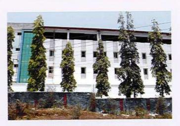
72 bedded Girls Hostel for Dr. B.R. Ambedkar Institute of Technology at Dollygunj is nearing completion. Hostel is RCC framed Triple storied building designed for earthquake resistance requirement conforming to Zone-V.
