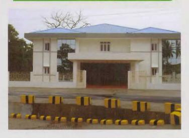
Office building for Archive has been completed within sanctioned amount during September 2013. This building will add to the Administrative Infrastructure. It has plinth area of 1602 Sqm. It is an Earthquake Resistant Double storied RCC framed structure equipped with Modern Fire Alarm system to prevent any untoward accident. Interior has been planned keeping in view optimum availability of space for accommodating records.
